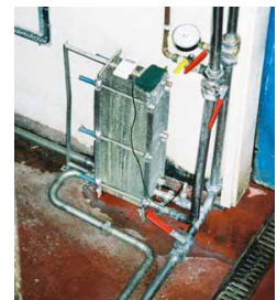
The wort chiller. Plate and frame for those of you who care.
